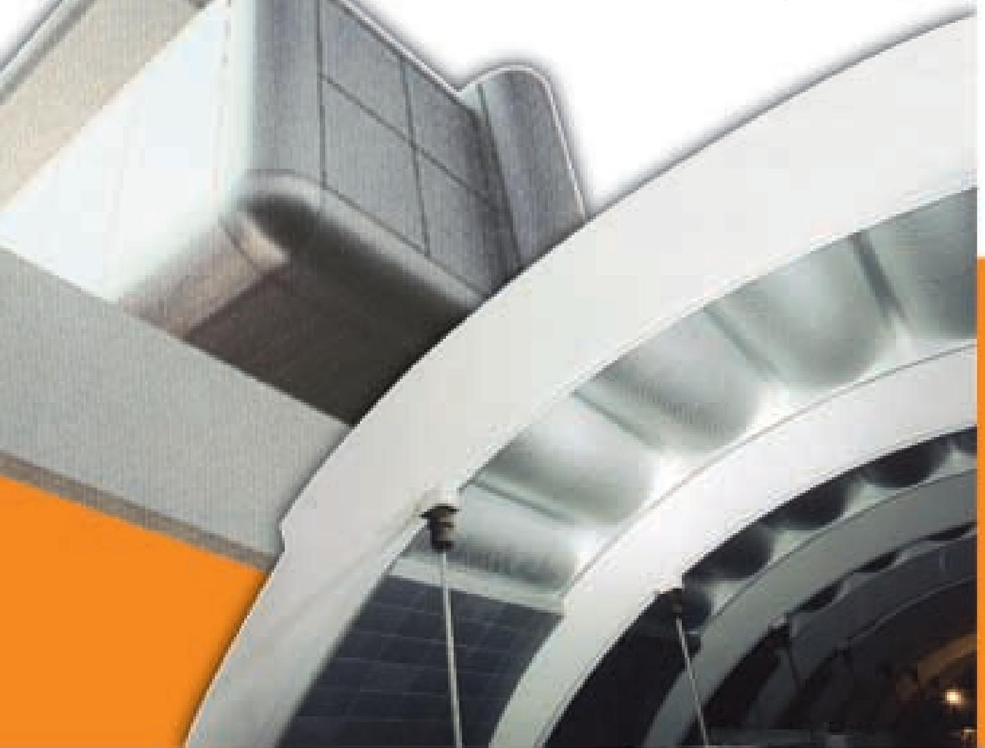
WINDY® is the Novelis brand name for its aluminium coils which have been pre-painted with polyamide paints. WINDY® is used in the building industry, especially in facade cladding, but also in windows frames. The excellent formability, the good bending behaviour of the product and the good resistance to UV rays make WINDY® particularly versatile and adaptable to different architectural solutions and industrial applications.
